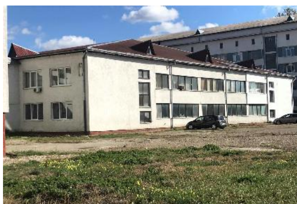
Figure 7 General view of the university building №9
