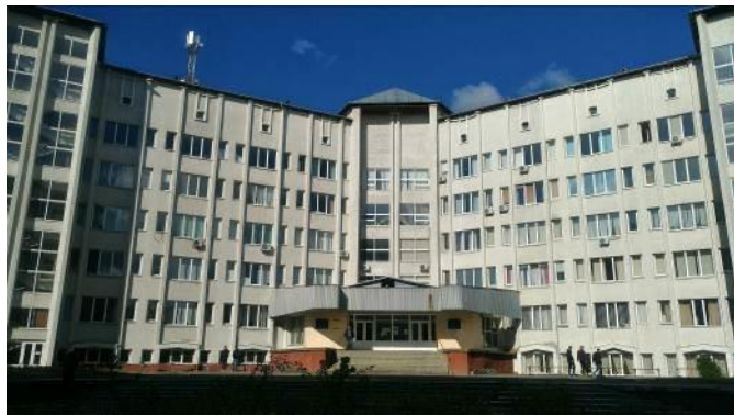
Figure 3 General view of the university building №1
