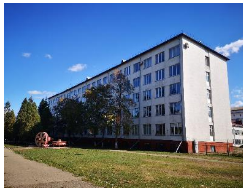
Figure 4 General view of the university building №4
