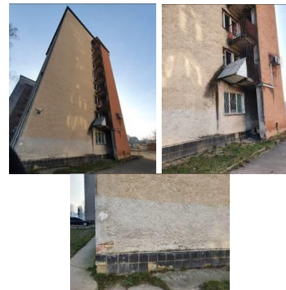
Figure 14 General view of the dormitory's №7 walls
