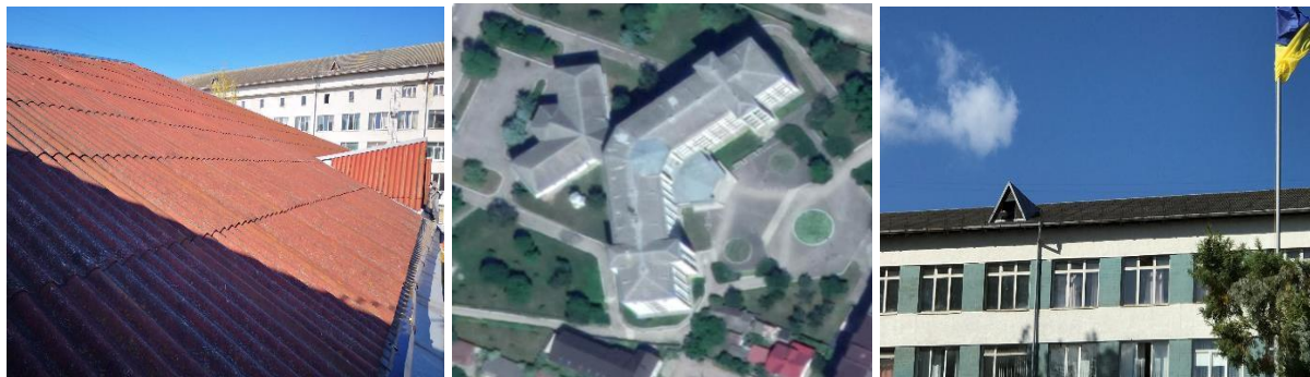
Figure 18 General view of the university buildings' roofs
