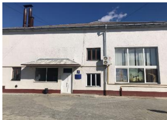
Figure 6 General view of the university building №7
