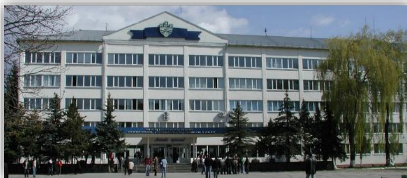
Figure 2 General view of the university building №0
