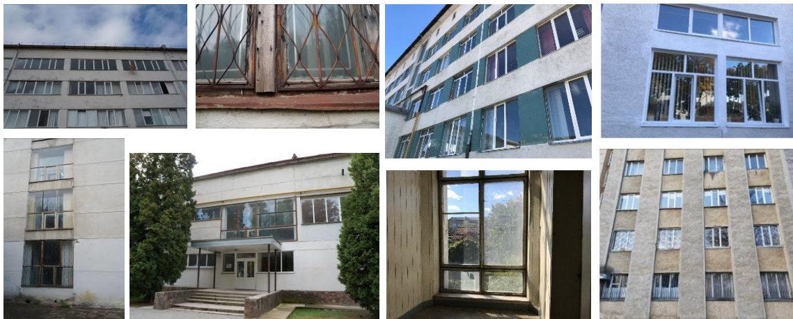
Figure 16 General view of the university buildings' windows
