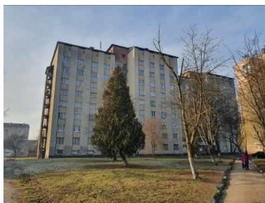
Figure 8 General view of the university dormitory №7
