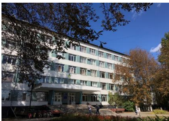
Figure 5 General view of the university building №5
